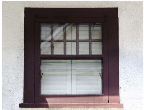
Image 3.4: hung-sash window with multi-pane (10) upper portion.
