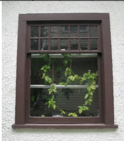
Image 3.5: hung-sash window with multi-pane (14) upper portion.
