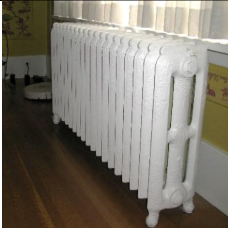
Image 7.5: example of one of the 10 cast iron radiators
