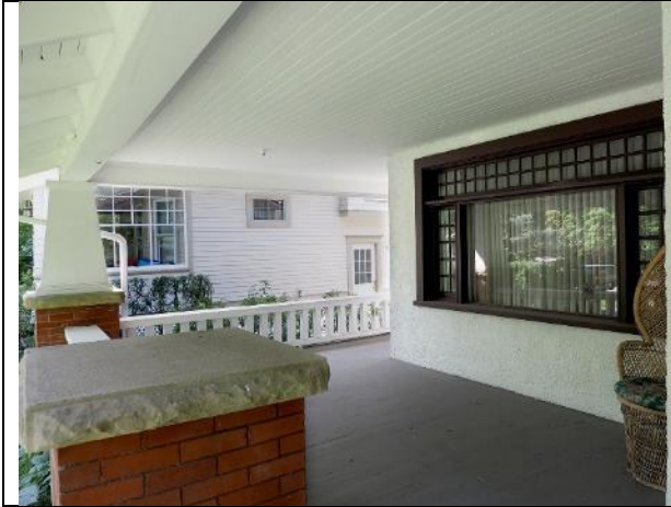
Image 1.3: detail showing open wrap around porch with with wooden tongue-and-groove ceiling; plain, painted-wood porch balustrade; tapered and paneled columns on brick (stretcher-bond) and sandstone piers; brick stairway pedestals with sandstone caps
