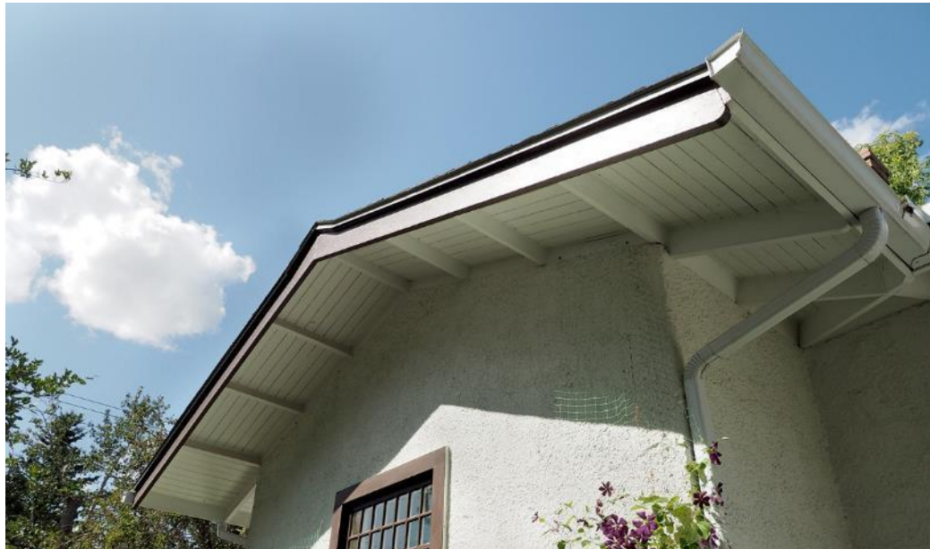
(Image 5.2: example of deep eaves with tongue-and-groove soffits with exposed plain rafters on remainder of building facades)
