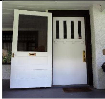
Image 1.6: Painted-wood slab front door with projecting band with brackets, 4 vertical lights
