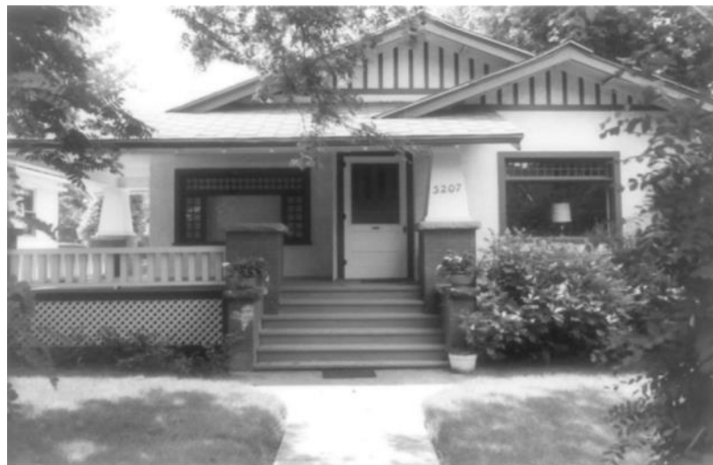
(Image 1.2: Historic view of east façade, 1983)
