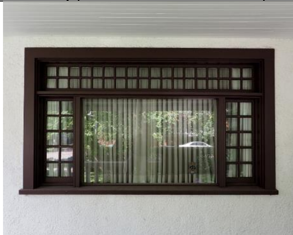
Image 1.5: three-part window comprising side casements with multiple panes (10 each), multi-pane (36) upper portion and a center fixed-pane.
