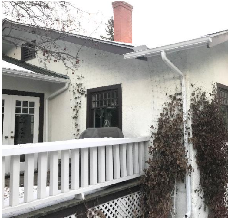
(Image 4.1: Oblique view of west façade)
