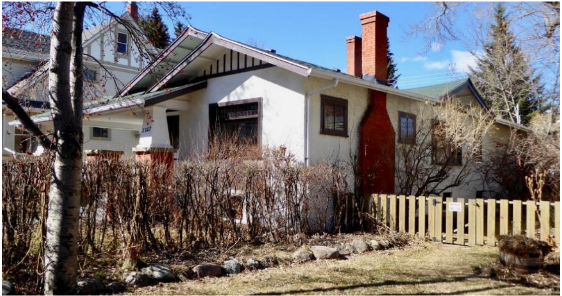
(Image 2.1: Oblique view of the north façade)
