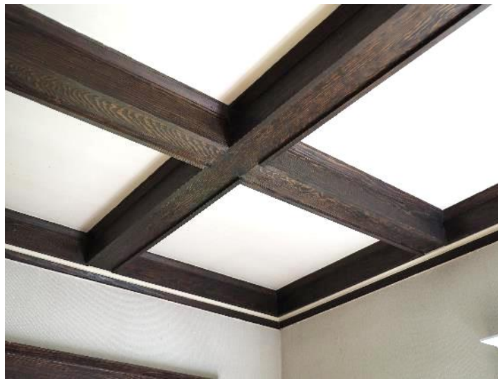
(Image 7.1: example of the wood ceiling beams)
