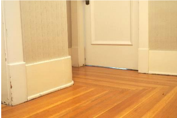
Image 7.3: example of the deep baseboards
