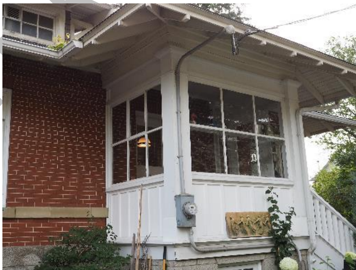
(Image 4.2: Enclosed porch trimmed with wooden paneling; wooden balustrade; six-lite windows)
