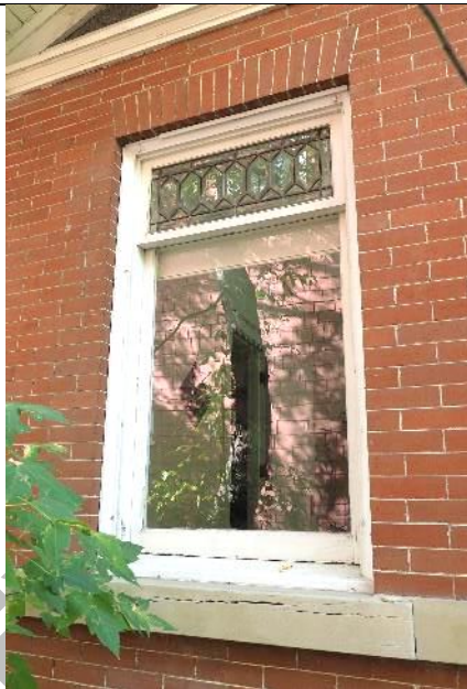
Image 2.5: Example of three of the five hung units with decorative beveled glass transoms
