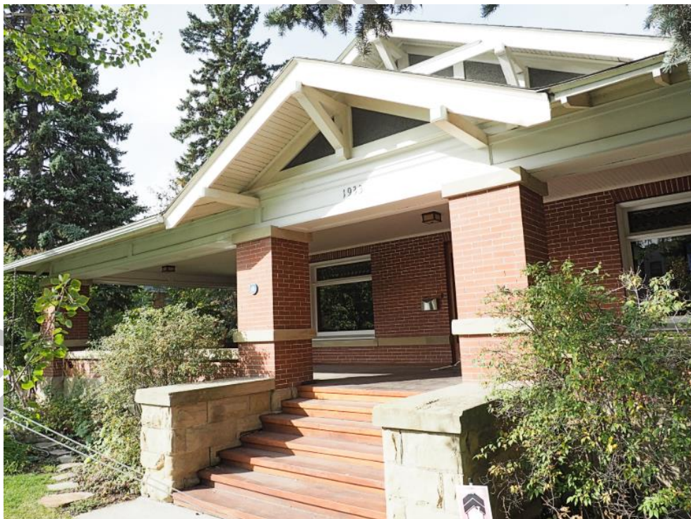
Image 1.3: Detail showing porch beam woodwork, brick posts with sandstone bands and caps; stairway pedestals clad with rock-face finish sandstone and sandstone caps
