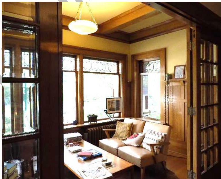
(Image 7.1: View into sun room with wood paneling, wood beams; wood room partition and French doors, both with beveled glass)
