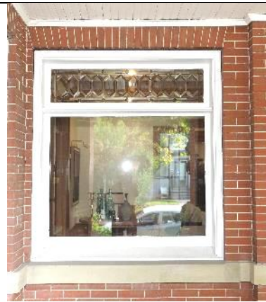
Image 3.8: One of two matching hung units both with decorative beveled glass transoms
