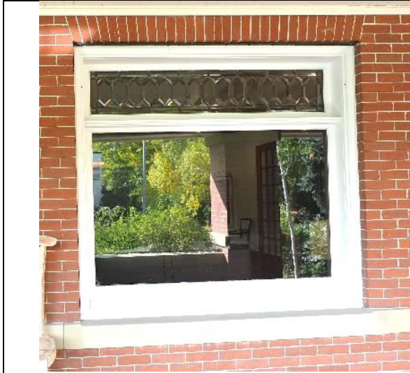
Image 1.4: Southernmost fixed pane unit with decorative beveled glass transoms
