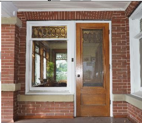
Image 3.7: Side entrance wood door flanked by a window, both with decorative beveled glass transoms; wood screen door
