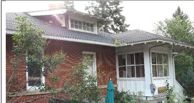
Image 5.3: West dormer with window; porch extension roof with exposed rafter tail ends
