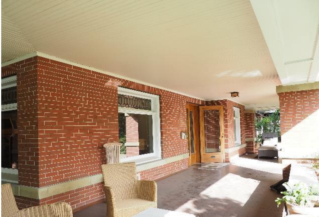
(Image 1.2: View looking northwest at the open wrap around porch with wooden tongue-and-groove ceiling; continuous sandstone band)
