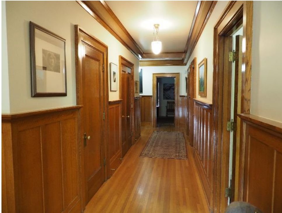
(Image 7.2: Central hallway with wood wainscoting; example of the wood doors, trim and baseboards; example of the oak flooring)
