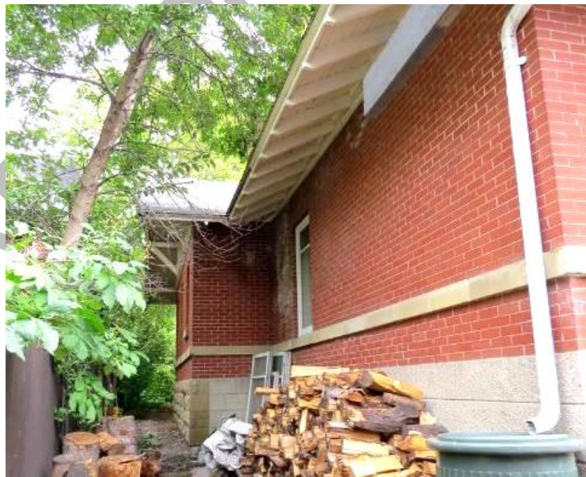
(Image 2.2: Oblique view of the north façade, looking east)
