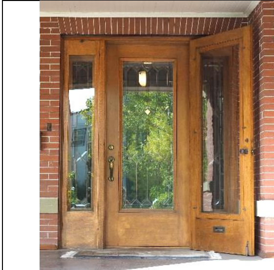
Image 1.6: Wood front door flanked by sidelites with decorative beveled glass; wood screen door
