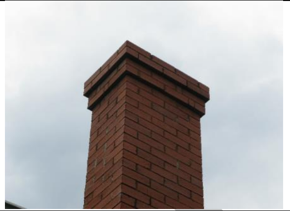
Image 2.5: detail of the chimney corbelled cap
