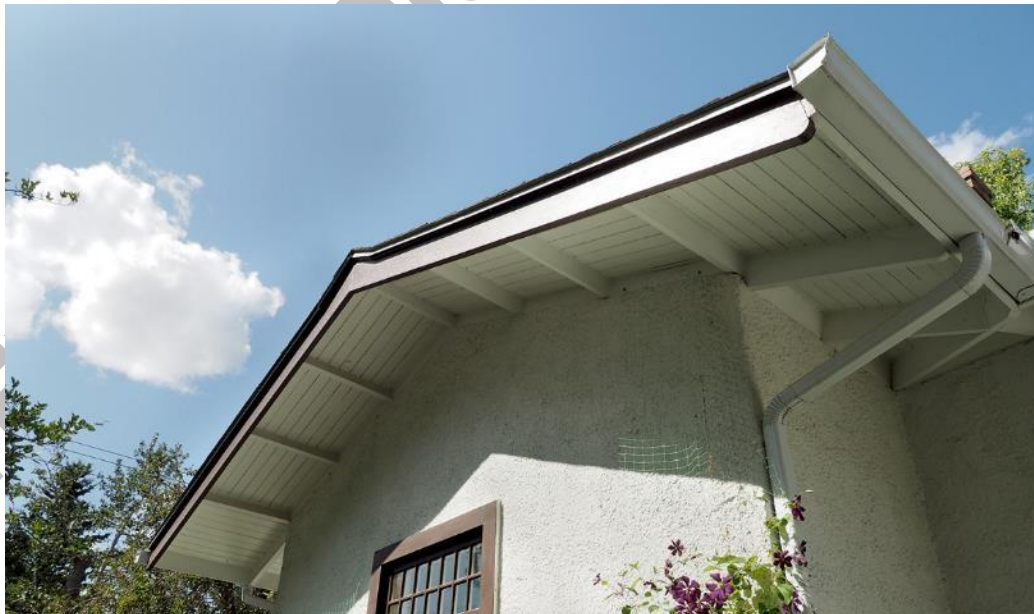
(Image 5.2: example of deep eaves with tongue-and-groove soffits with exposed plain rafters on remainder of building facades)
