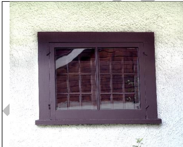
Image 2.2: detail showing one of the two matching windows flanking the fireplace chimney, comprised of two casement windows with multiple panes (9 each)
