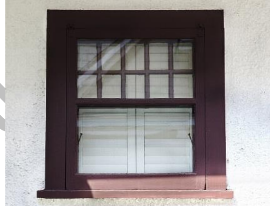
Image 3.4: hung-sash window with multi-pane (10) upper portion.
