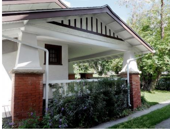
(Image 3.2: south portion of open wrap around porch with with wooden tongue-and-groove ceiling; plain, painted-wood porch balustrade; tapered and paneled columns on brick and sandstone piers)
