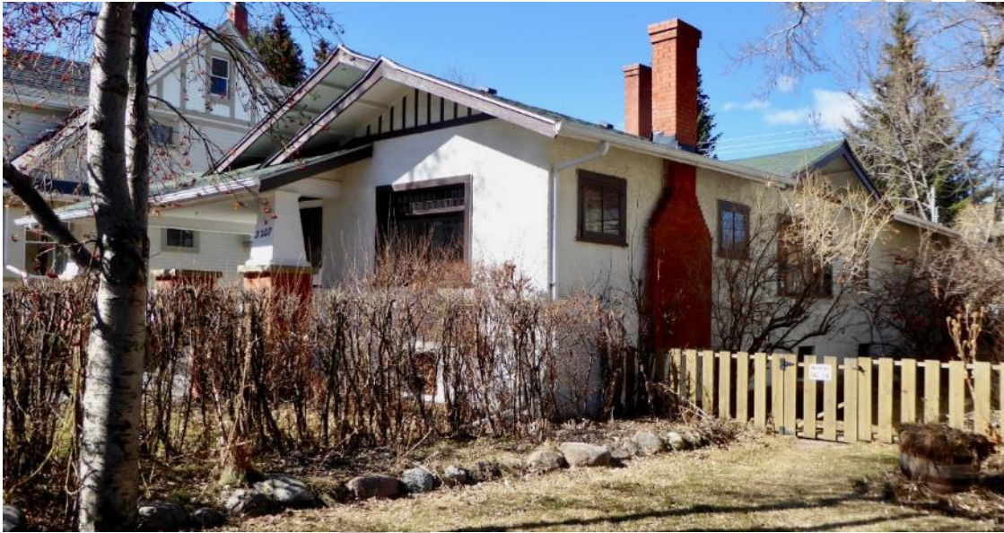
(Image 2.1: Oblique view of the north façade)
