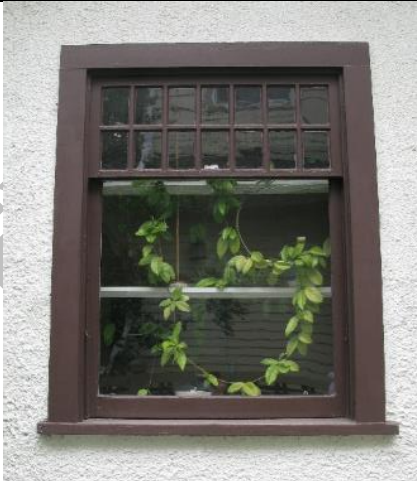
Image 3.5: hung-sash window with multi-pane (14) upper portion.
