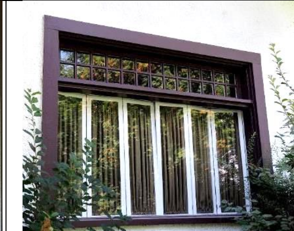
Image 1.4: fixed-pane picture window with multi-pane (26) upper portion.
