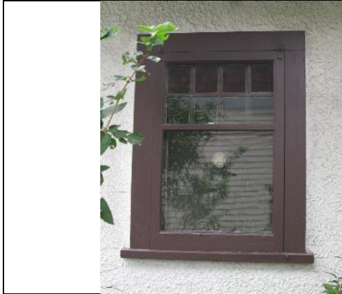
Image 2.4: hung-sash window with multi-pane (8) upper portion.
