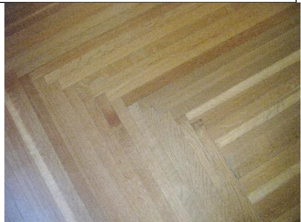
Image 7.8: detail of the white-oak plank floors laid with alternate-direction border
