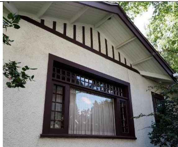
Image 2.3: three-part window comprising side casements with multiple panes (10), multi-pane (36) upper portion and a center fixed-pane.
