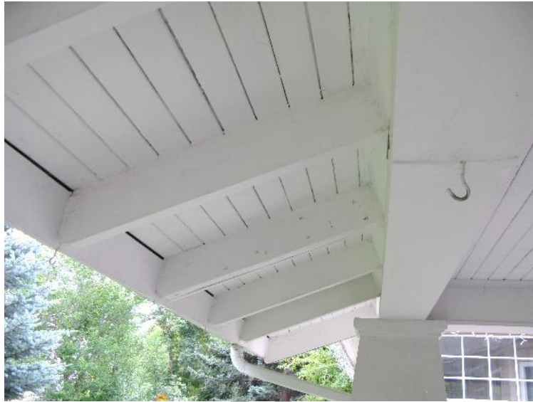
(Image 5.1: example of deep eaves with tongue-and-groove soffits with exposed rounded-end rafters on east roof of wrap around porch)
