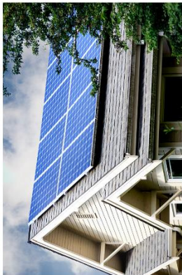
Photo: Solar panels to capture solar energy.
