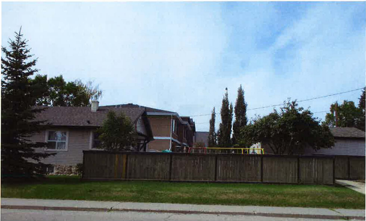
Photo 1b. LOC2019-0029 Property. Side view, showing neighbouring homes and back gardens.
