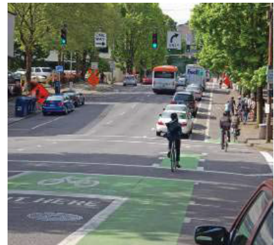
Bike box and buffered cycle track lane
