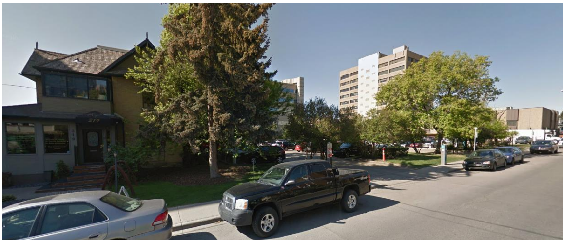
DC Site 2: 319 - 15 Avenue SW and 1520 4 Street SW (receiver)
