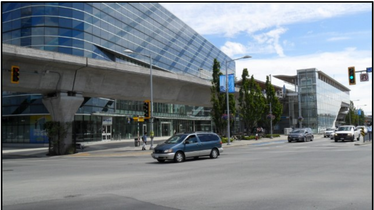
Figure 2: Canada Line Station in Richmond
