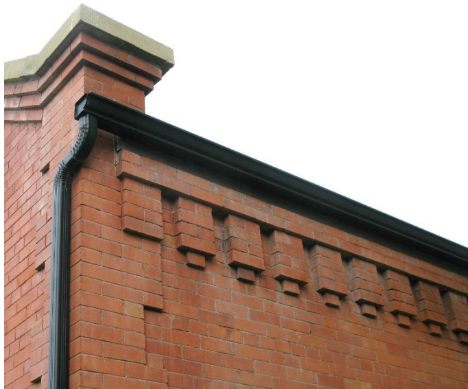
(Image 2.3: example of the brick corbelled cornice with corbelled modillions at roof line, and the projecting quoins at building corners)
