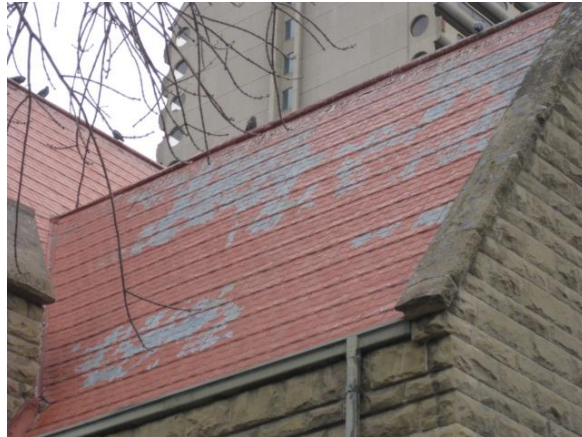
(Photo 2.7: smooth sandstone coping of gables and example of the metal roofing )
