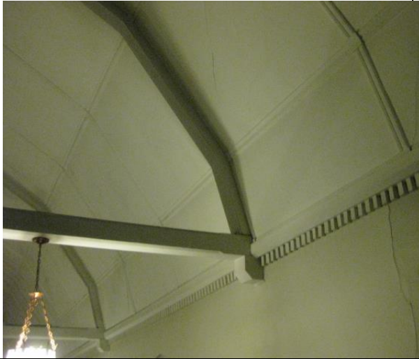
(Photo 3.9: ceiling features including barrel-vault nave, exposed timber trusses and dentil mouldings (nave))
