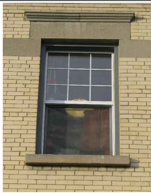
(Image 1.3: example of the sandstone detailing lintels and stringcourse on third storey windows)
