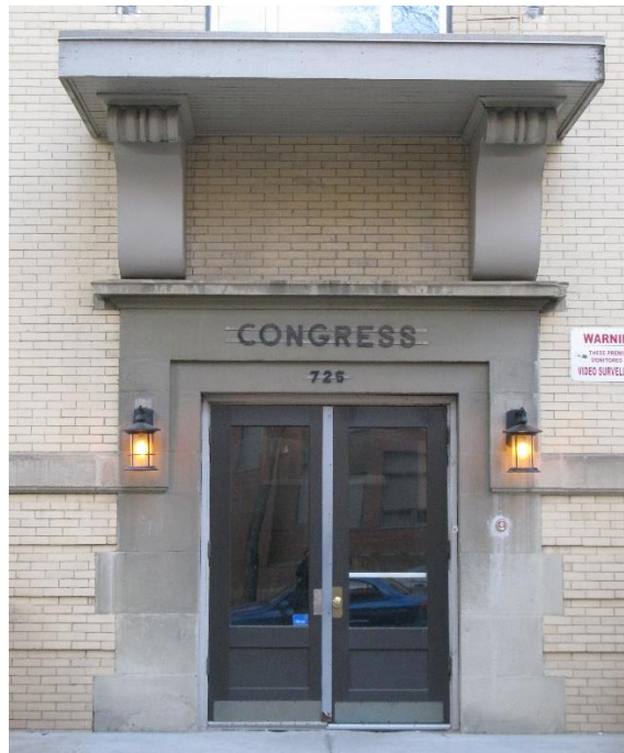
(Image 1.4: The sandstone “blocked” doorway surround intersected by sandstone stringcourse and foundation level brickwork relief in horizontal bands. Portion of the second-storey balcony with classic corbels remains)
