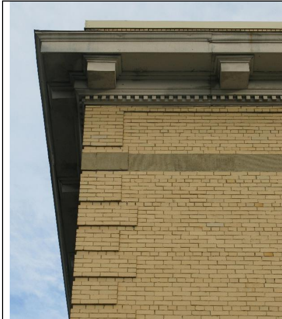
(Image 1.2: examples of the buff colored brick quoins on North Façade corners and the pressed-metal cornice in block-modillion and dentil design)
