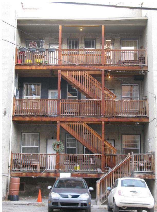
(Image 3.2: South Façade fenestration and the inset-open three storey wooden porch with stairs from grade to third floor)
