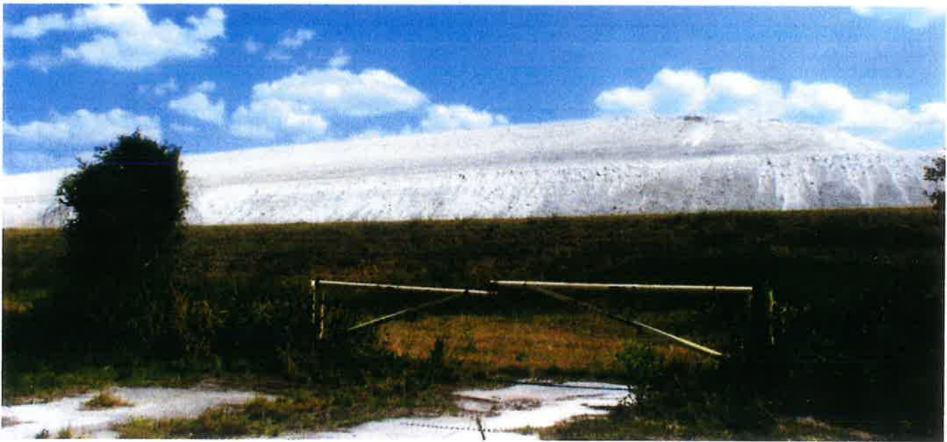
Phosphogypsum stack located near Fort Meade, Florida. These contain the waste byproducts of the phosphate fertilizer industry.
