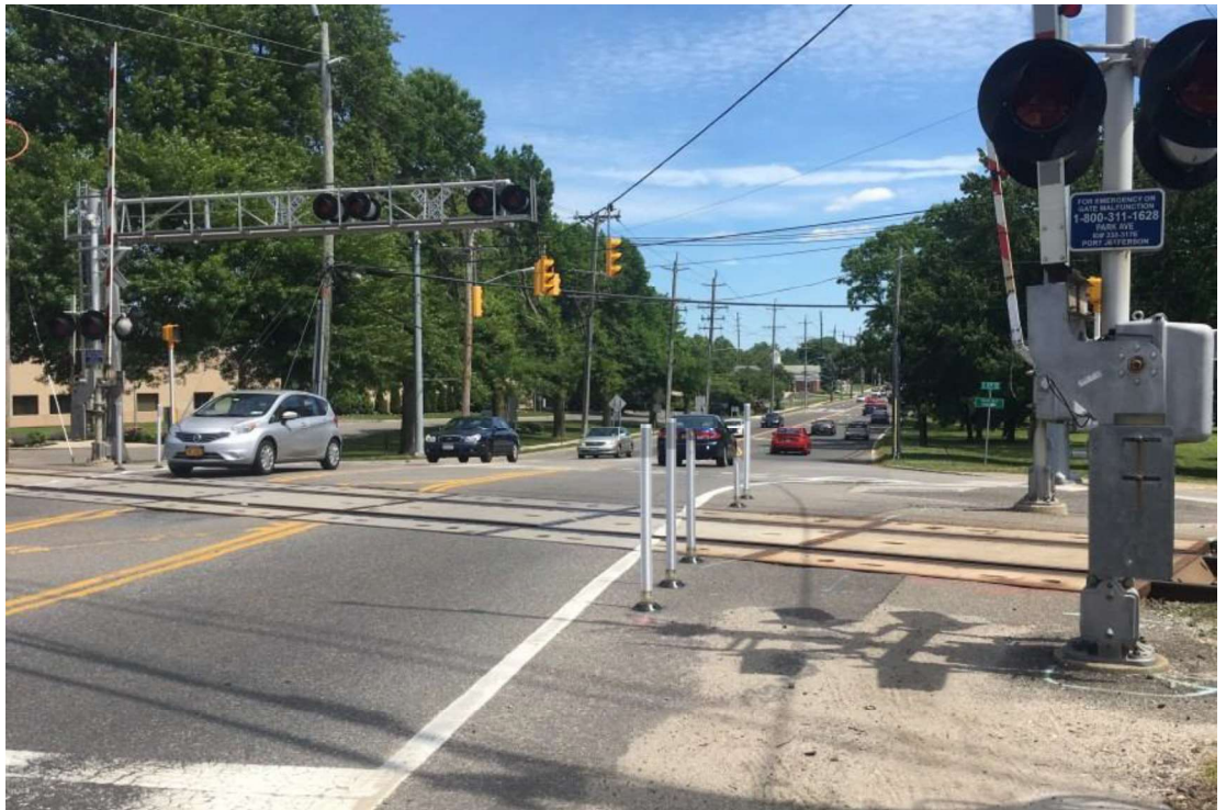
Figure 10-4 Crossing Edge Markings on LIRR (Huntington NOW)
