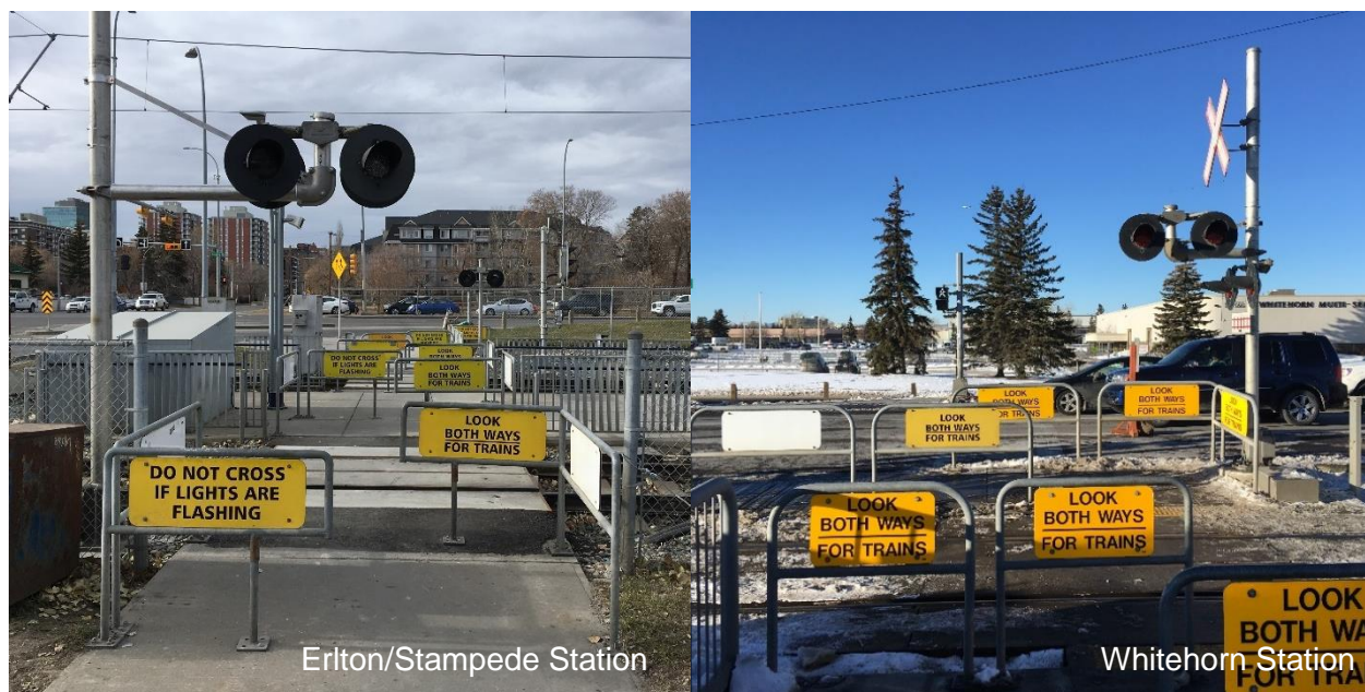
Figure 3: Flashing lights lowered and cantilevered out to directly face pedestrians.
