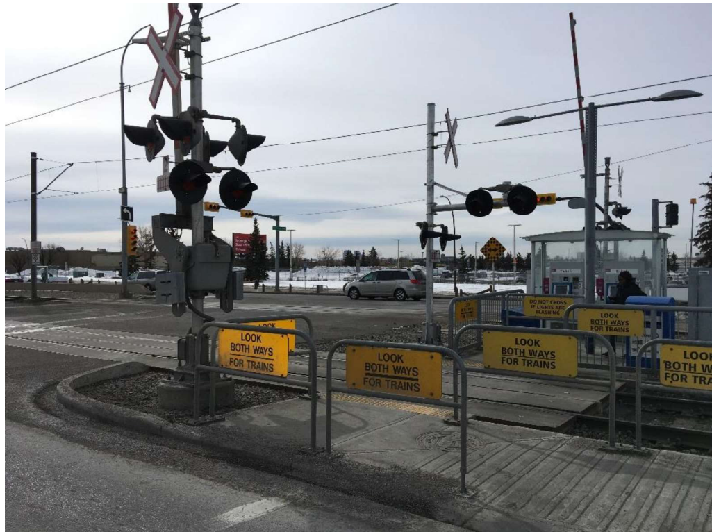
Figure 6-3 Revised Crossing Signals at Whitehorn Station (Calgary Transit)
