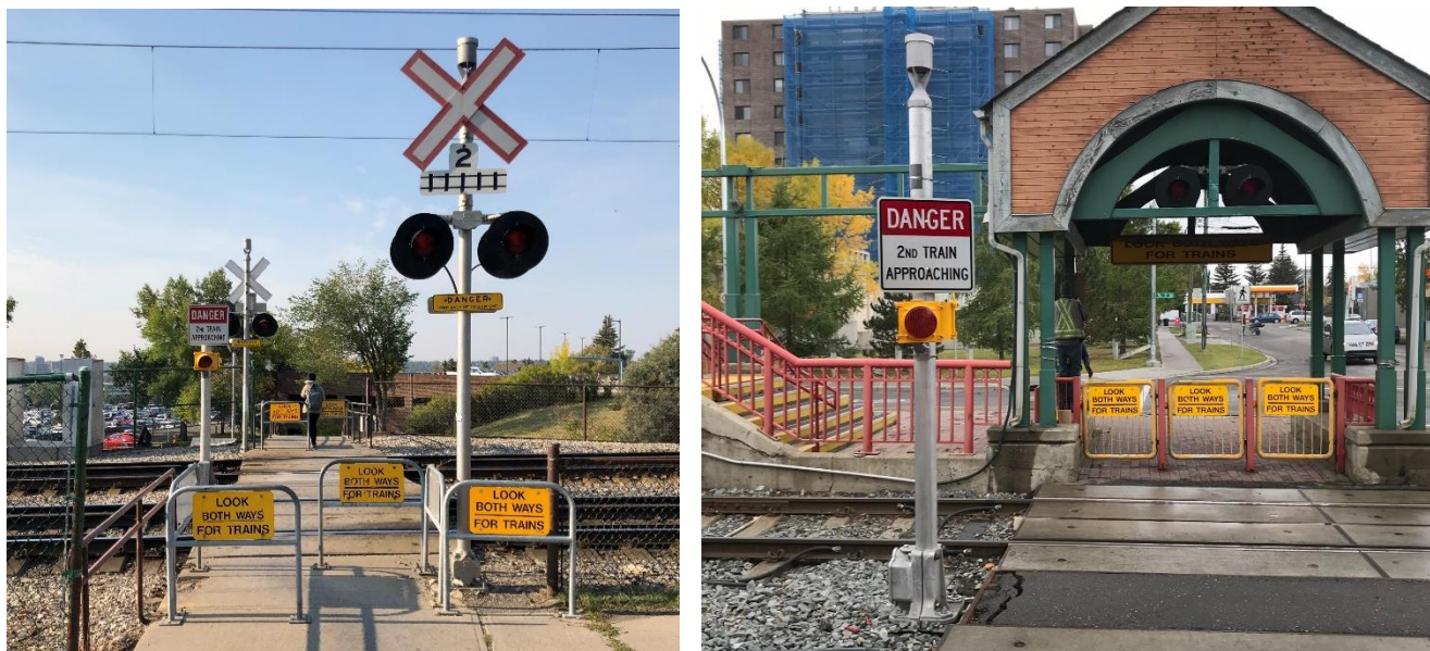
Figure 5: Second Train Lights at SAIT Campus Crossing (left) and Sunnyside Station Crossing (right)
