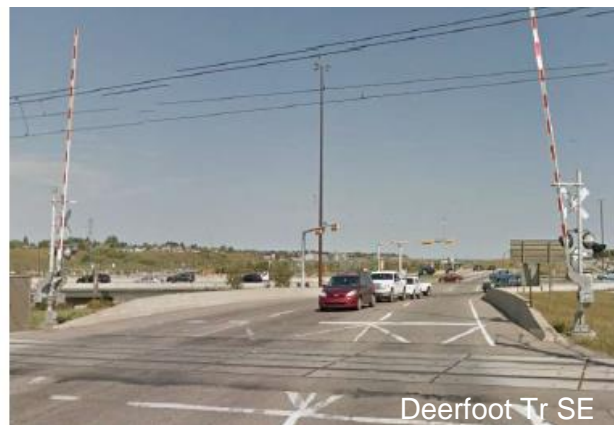
Figure 1: (left) flashing lights, bells and besteads; (middle) automatic pedestrian gate arm, flashing light and bells; (right) automatic vehicle gate arms
