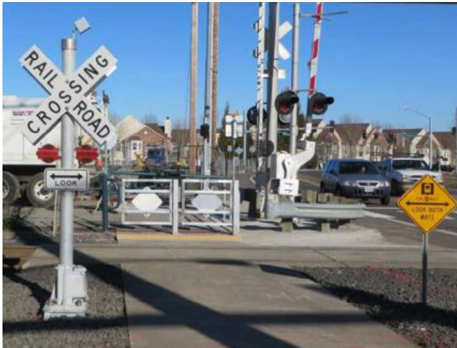
Figure 7-4 Smaller Scale Pedestrian Flasher in Portland (Fitzpatrick)
