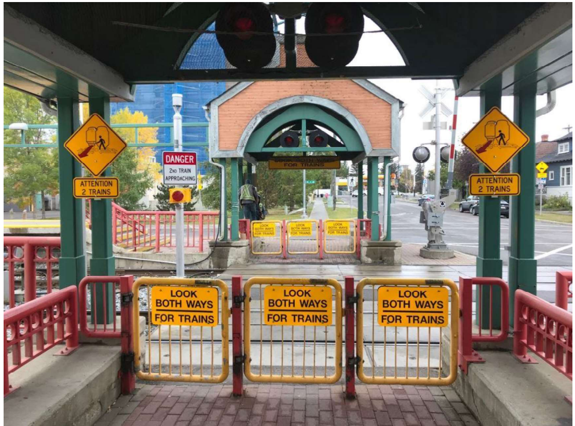
Figure 6-2 Second Train Warning Signage at Sunnyside Station (Calgary Transit)
