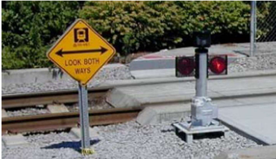
Figure 7-3 "Portland Style" Pedestrian Flasher
