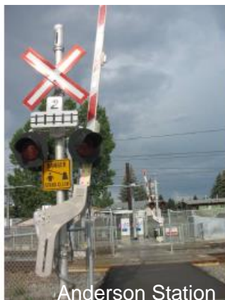
Figure 1: (left) flashing lights, bells and besteads; (middle) automatic pedestrian gate arm, flashing light and bells; (right) automatic vehicle gate arms
