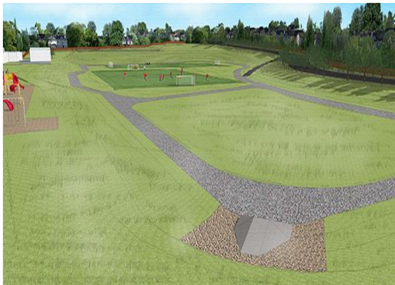
THE BRAESIDE DRY POND WILL GREATLY REDUCE FLOODING DURING EXTREME RAIN EVENTS NEAR SOUTHLAND DRIVE SW AND BRAESIDE DRIVE SW.
