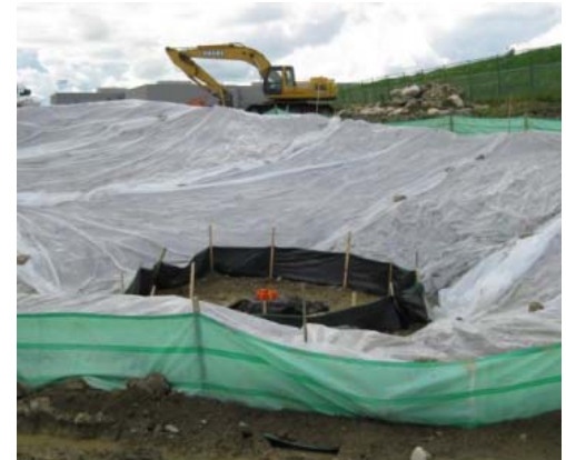
FIGURE 4.9 EROSION AND SEDIMENT CONTROL DURING CONSTRUCTION HELPS PROTECT THE WATERSHED AND STORM INFRASTRUCTURE.
