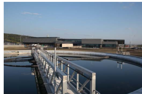
FIGURE 4.2 PINE CREEK WASTEWATER TREATMENT PLANT
