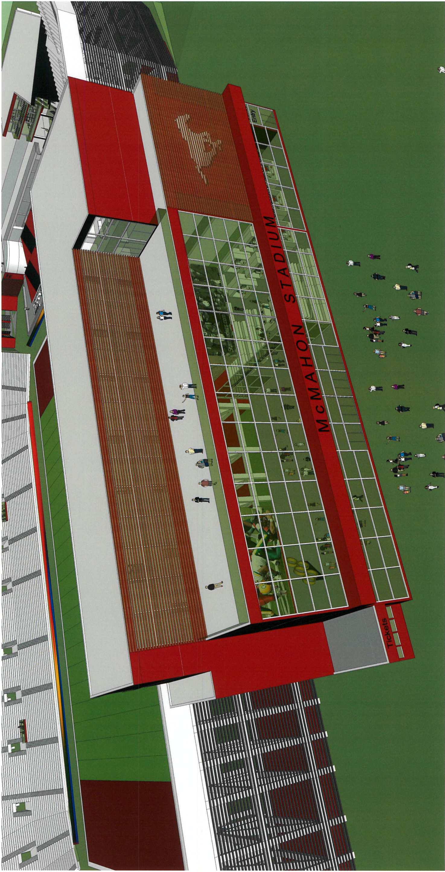
View of the new 48,000 square-foot Main Entrance pavilion as seen from the air from the east. The new addition features a new grand lobby, two upper concourse levels and two levels of corporate suites including an owner's suite
