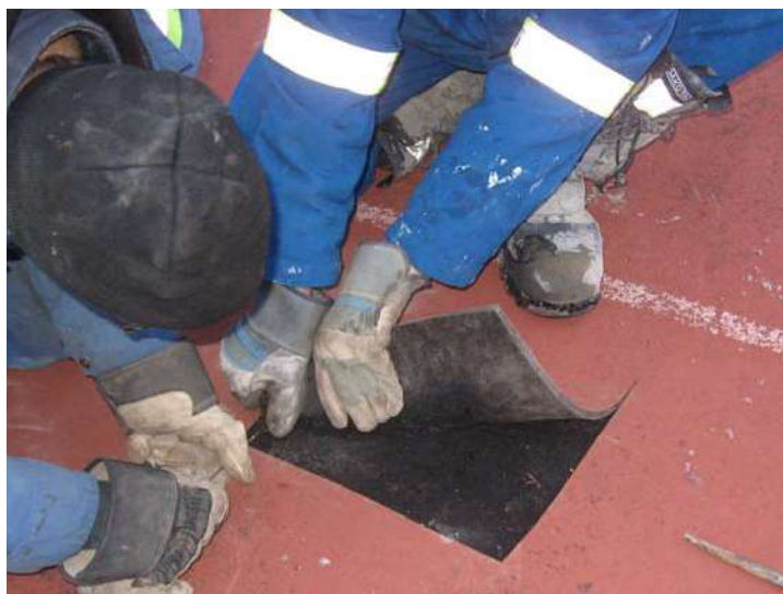
Photo 1: Ripping the surface material at BH02 before augering
