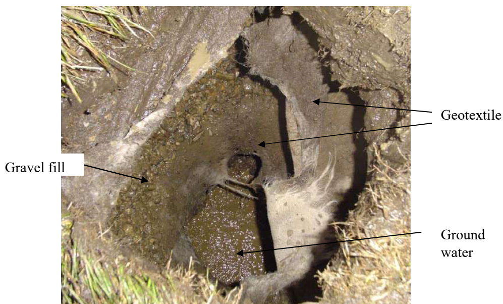
Photo 5: BH04 after vacuum excavation
