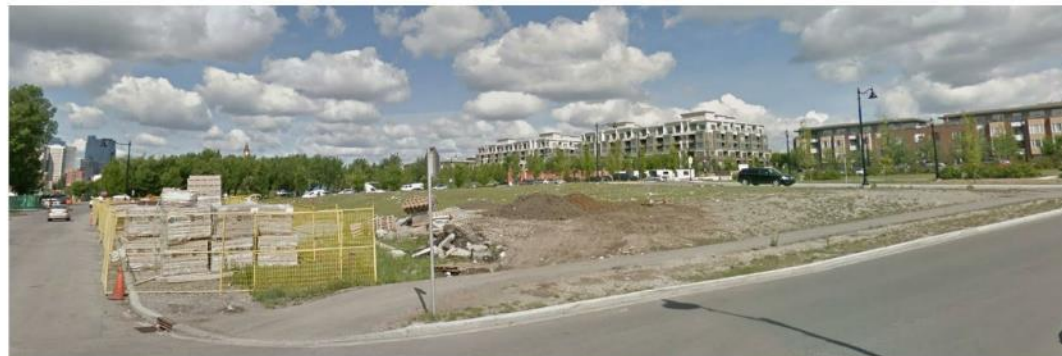
VIEW 3 : SOUTHEAST VIEW OF SITE
