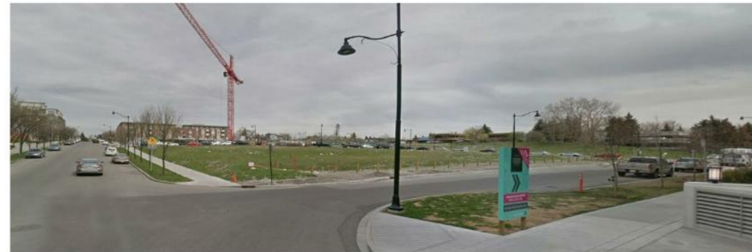
VIEW 2 : SOUTHWEST VIEW OF SITE
