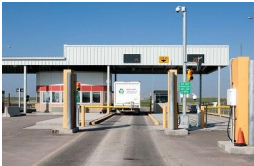
Photo: Shepard Waste Management Facility scale house
