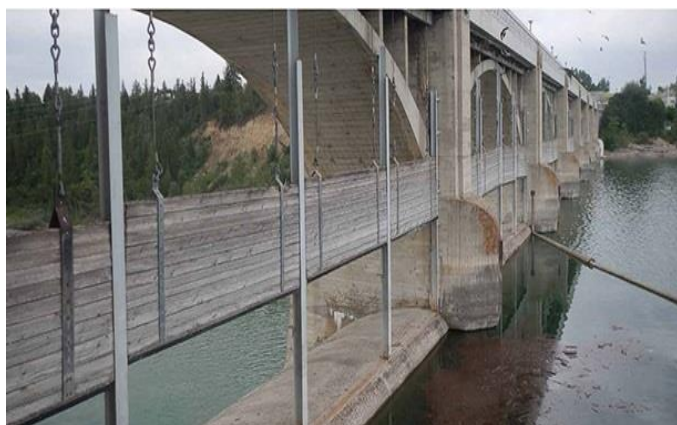
UPGRADES AT THE GLENMORE DAM INCLUDE REPLACING THESE STOP LOGS WITH AUTOMATED STEEL GATES FOR IMPROVED WATER STORAGE AND FLOOD MITIGATION CONTROL.
