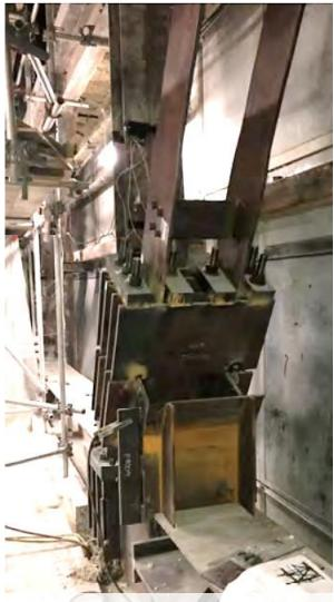
Truss 'A' Modification Completed with "Stiffeners"
