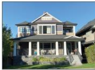
Recessed upper deck
