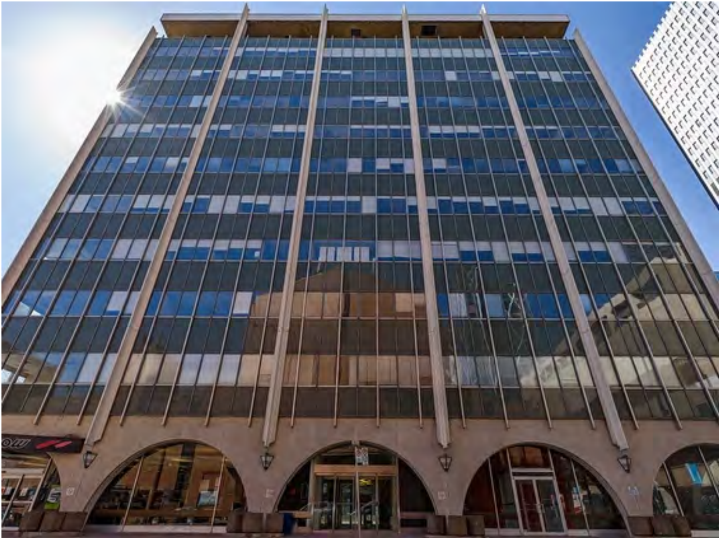
HAT @ Arts Common, one of the first three approved projects of the Downtown Calgary Development Incentive Program. Azin Ghaffari/Postmedia
