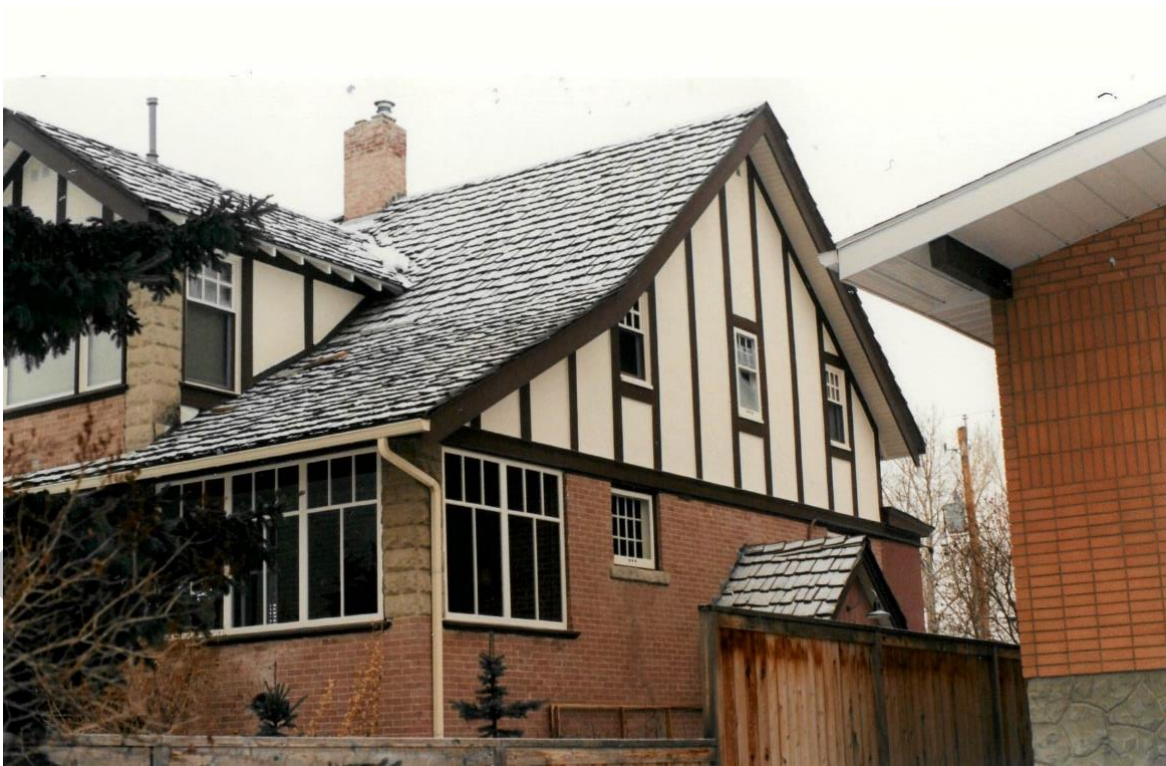
(Image 2.3: photo ca.1996, view of house from southeast)
