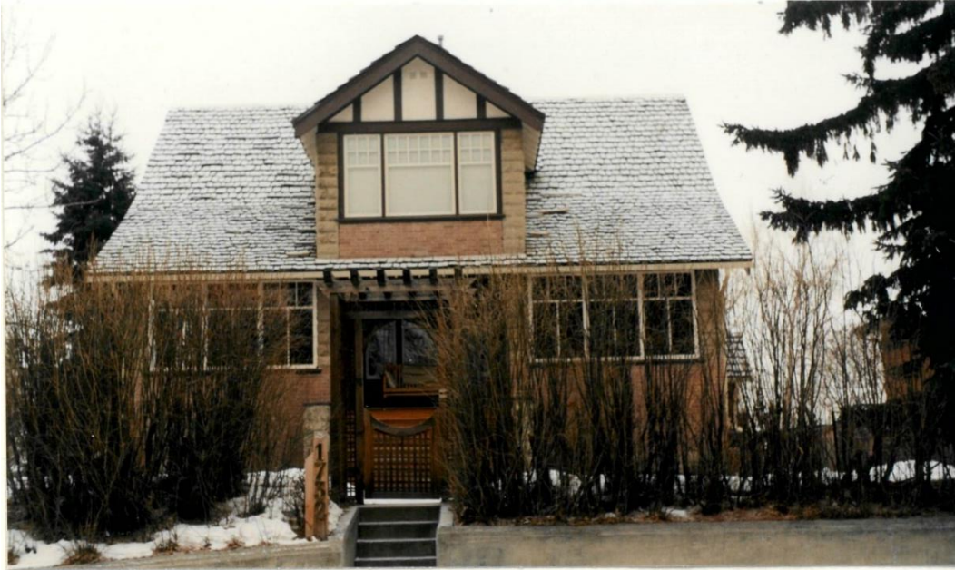
(Image 1.2: ca. 1996 photo showing south façade with original window assembly on second storey)
