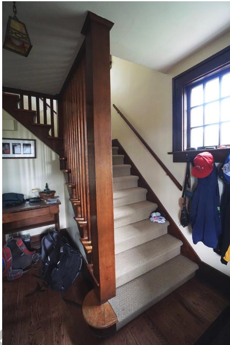
(Image 7.7: Quarter-turn closed staircase to second storey with Douglas fir stair rail, newel, and balustrade; example of a window casing)
