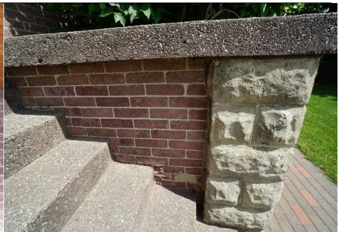
(Image 1.8: Detail showing exterior front stairs: walls of concrete bricks laid in stretcher bond and hollow rock-faced concrete blocks)
