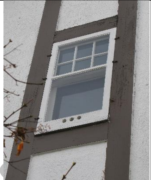
(Image 2.5: example of one of three 6-over-1 wood hung windows with flat heads and painted wood trim)
