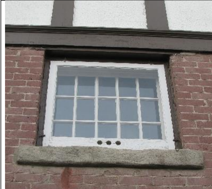
(Image 2.4: example of one of two 15-pane wood windows with concrete sills; continuous wood band with decorative trim)
