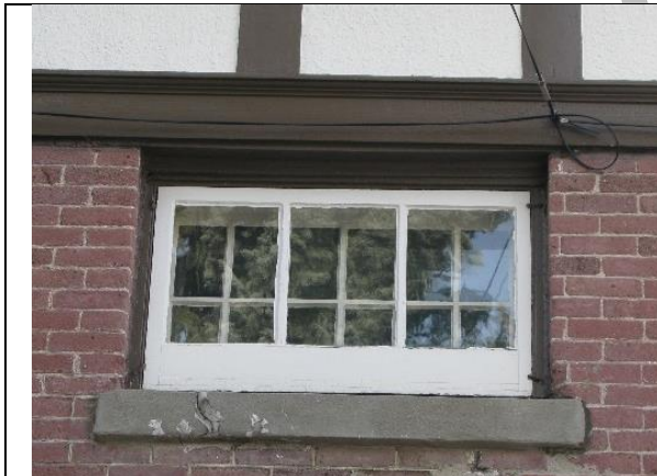
(Image 4.3: 12-pane wood window with concrete sill)
