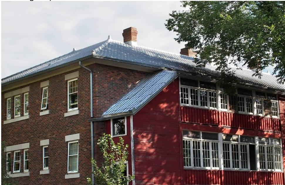
(Image #2.12 – North and east elevations, showing rear veranda/fire escape and galvanized Spanish metal roof tile)
