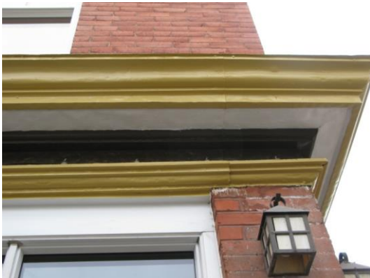
(Photo 1.3: A portion of the pressed-metal storefront cornice)
