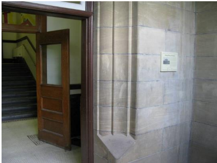
(Photo 6.1.09: First Floor - Main entrance porch and foyer showing ashlar sandstone wall finishes)
