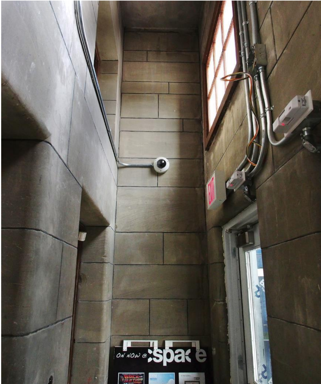
(Photo 6.1.11: First Floor - 'BOYS' side entrance showing outer foyer ashlar sandstone wall finish)
