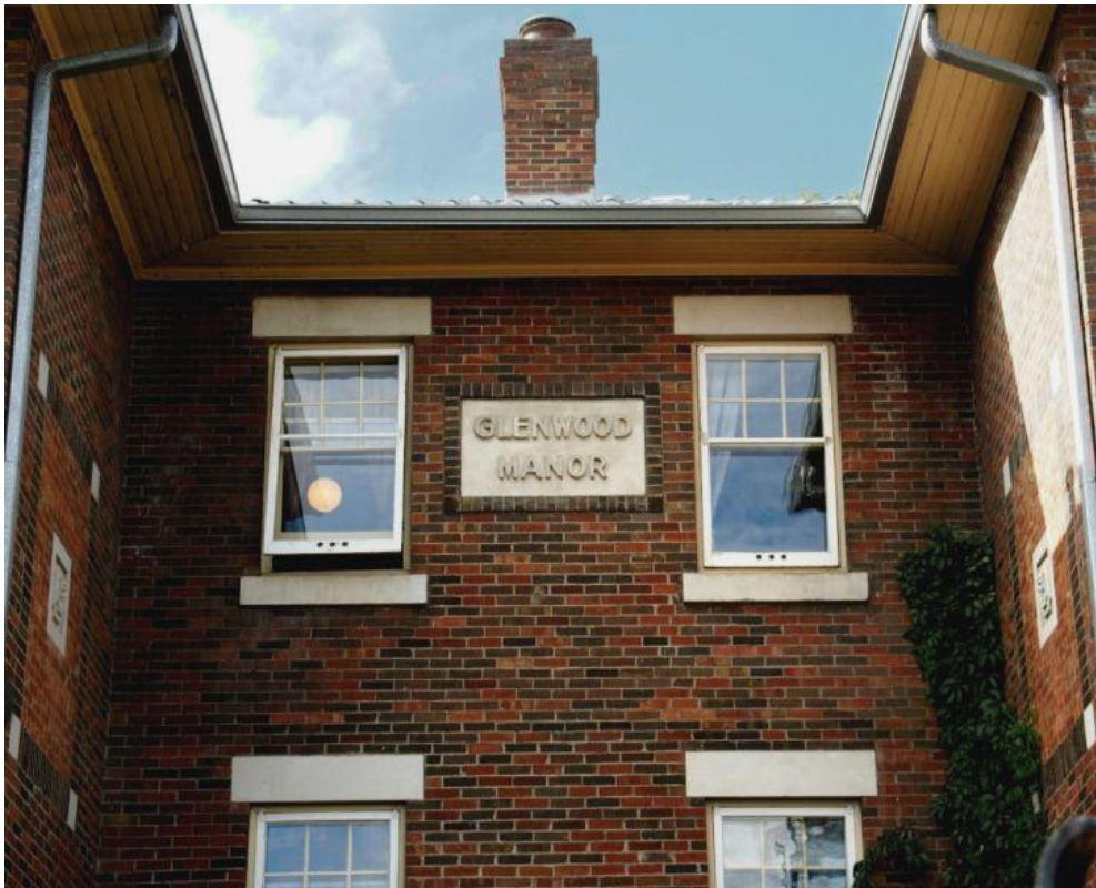
(Image #2.8 – Centre of u-shaped plan, showing deep eaves and wood soffits, GLENWOOD MANOR inset panel)
