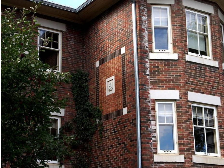
(Image #2.7 – Red-brick exterior in simple stretcher bond, concrete window sills and lintels and one of three decorative panels)
