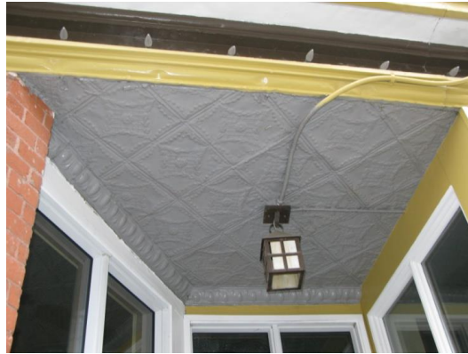
(Photo 1.4: A portion of the pressed metal ceiling in the central recessed entry bay)
