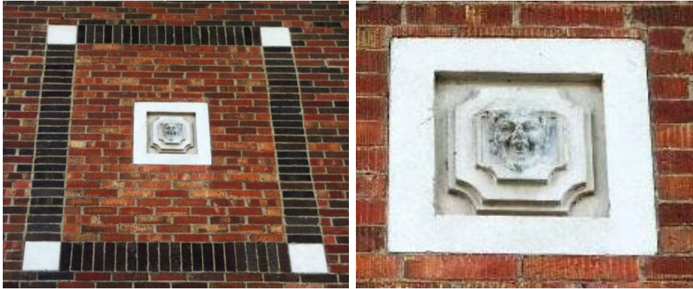
(Image #2.9 – Detail of decorative panel with inset art stone and dark brick surround)
