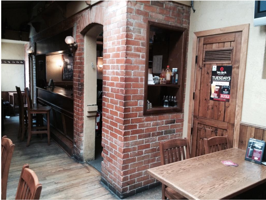
(Photo 10.1: The westerly brick wall – formerly the exterior west façade)
