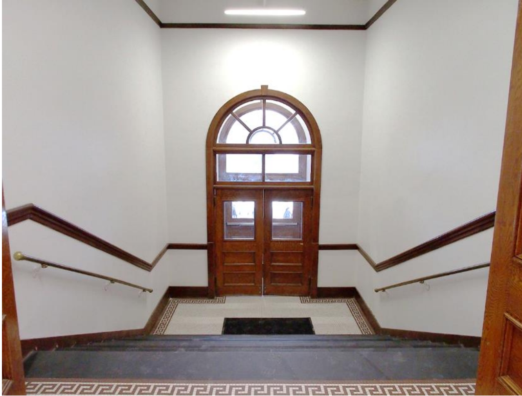
(Photo 6.1.08: First Floor – Main entrance foyer showing patterned porcelain flooring and interior doorway assembly with transom lights and fanlights)
