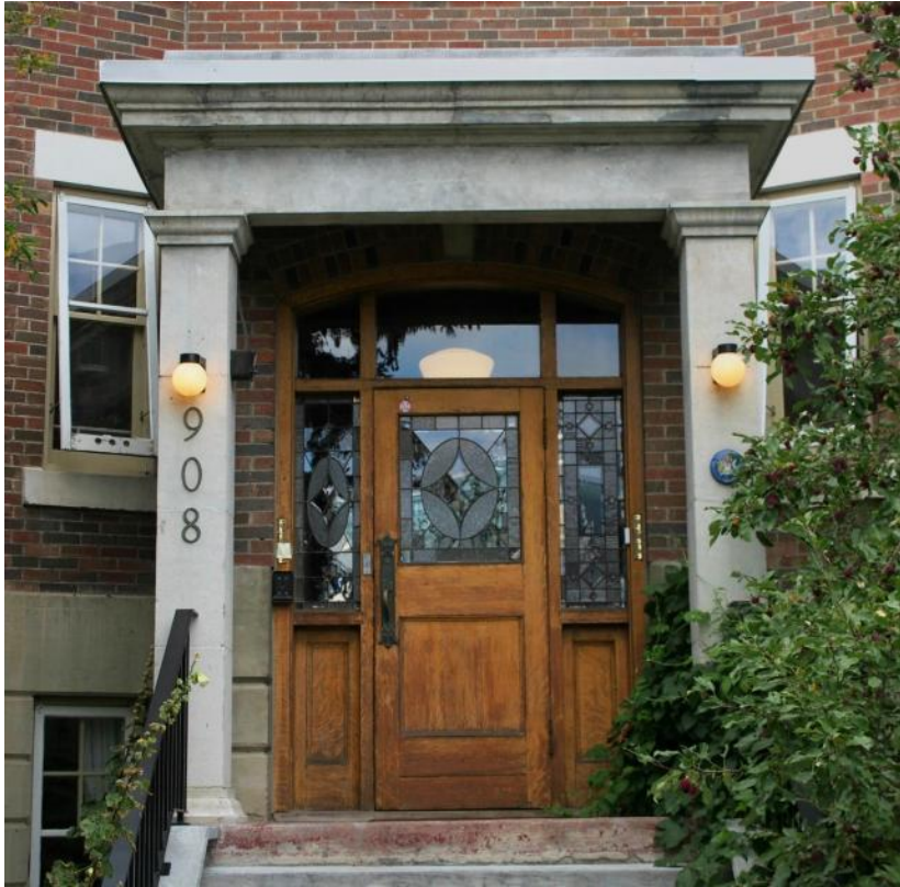
(Image #2.11 – Entry door and surround with transom configuration and leaded glass)
