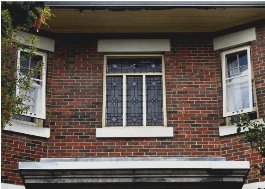
(Image #2.10 – One of two transom window arrangements with leaded glass)
