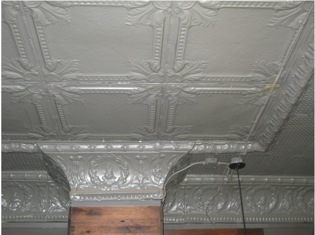
(Photo 5.1: Example of the pressed metal ceiling and cornice mouldings of the first-storey interior)
