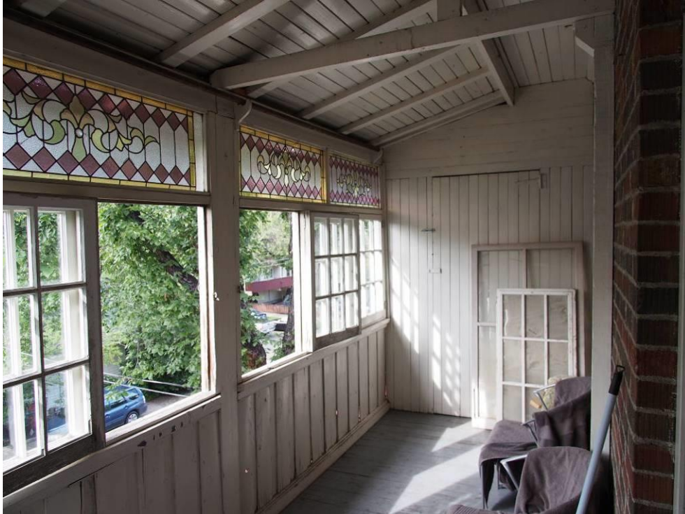
(Image #2.13 – Present form of rear veranda/fire escape showing plain balusters. Windows and interior configuration non-regulated)
