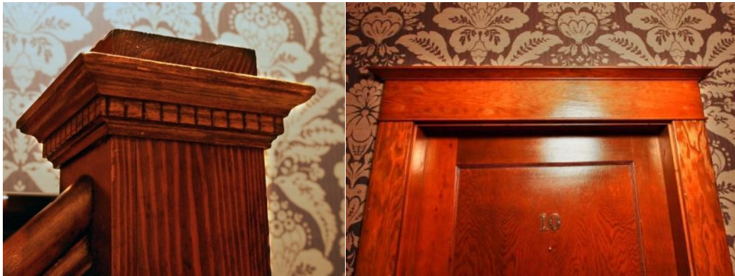
(Image #3.4 – Typical fir detailing on newel post and door casing)
