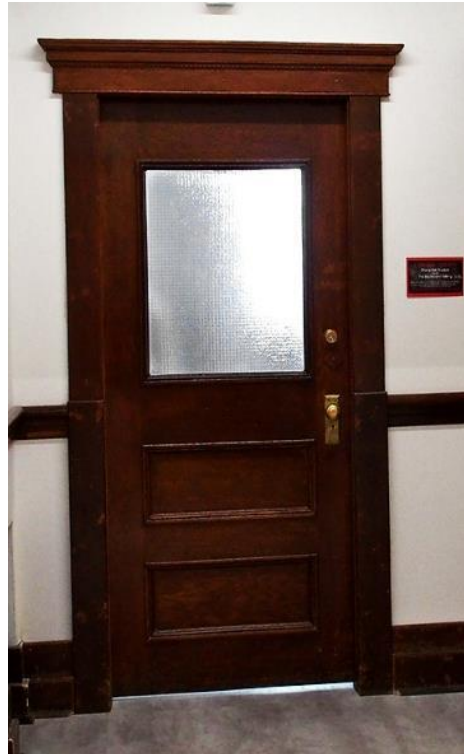
(Photo 6.1.07: An example of a paneled and glazed door and door casings common throughout the building)
