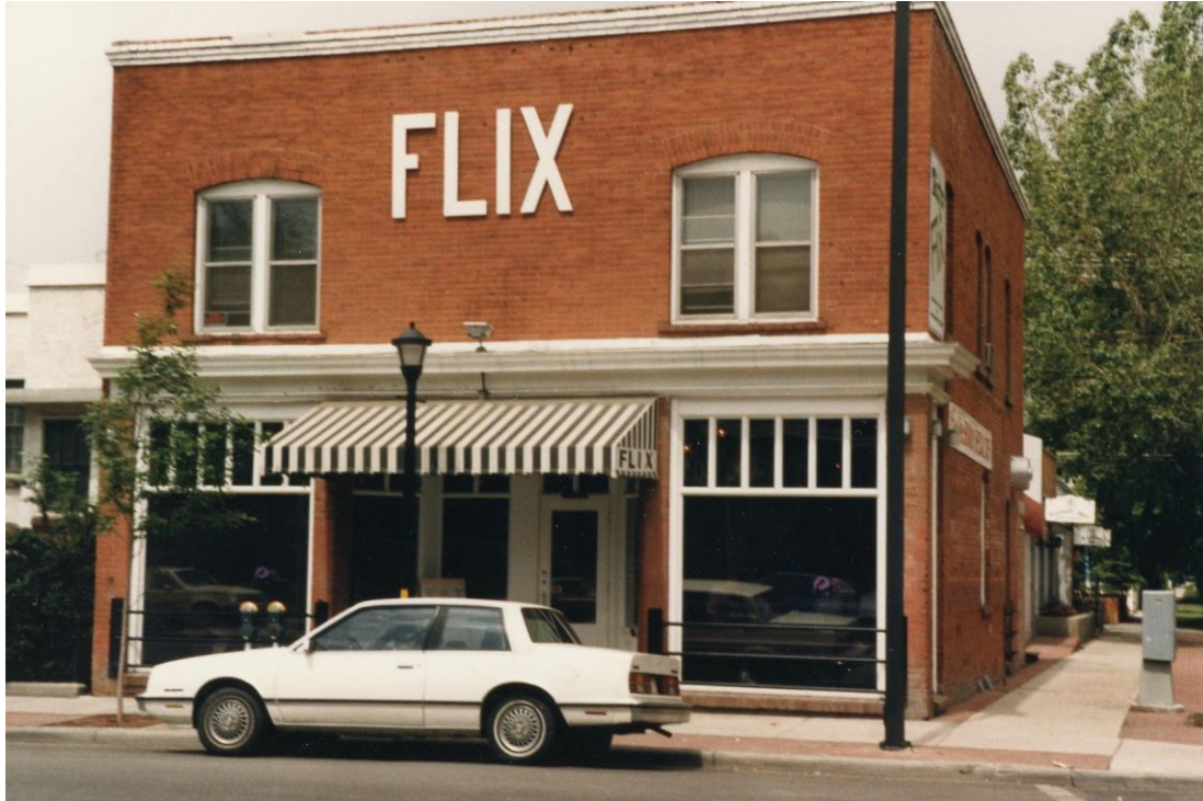
(Photo 1.2: 1985 photo showing south façade, including the historical appearance of the storefront, the corbelled roofline cornice, and brick window sills— courtesy Province of Alberta Heritage Survey Program 11-138 1985 P1)
