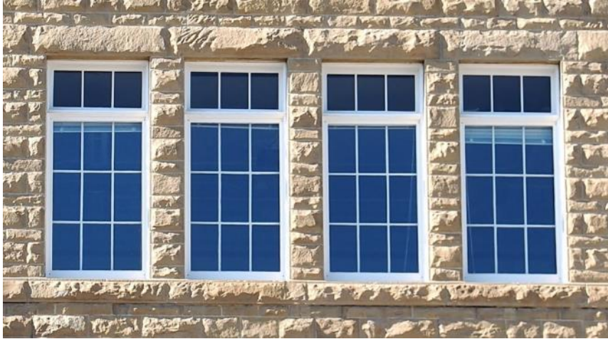
(Photo 1.4: An example of the wooden-sash, nine-pane windows with three-pane transom lights)
