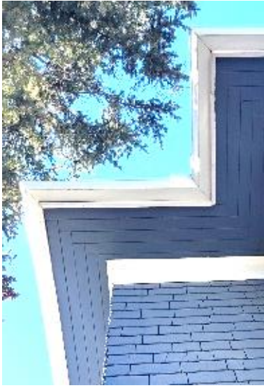
(Image 2.5: example of closed wooden tongue-and-groove soffits)
