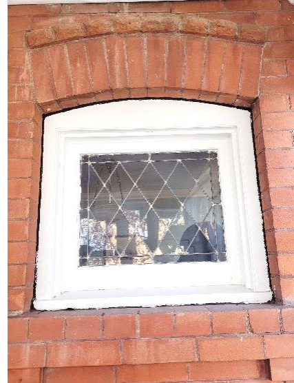
(Image 2.7: example of single sash window with decorative diamond patterned)
