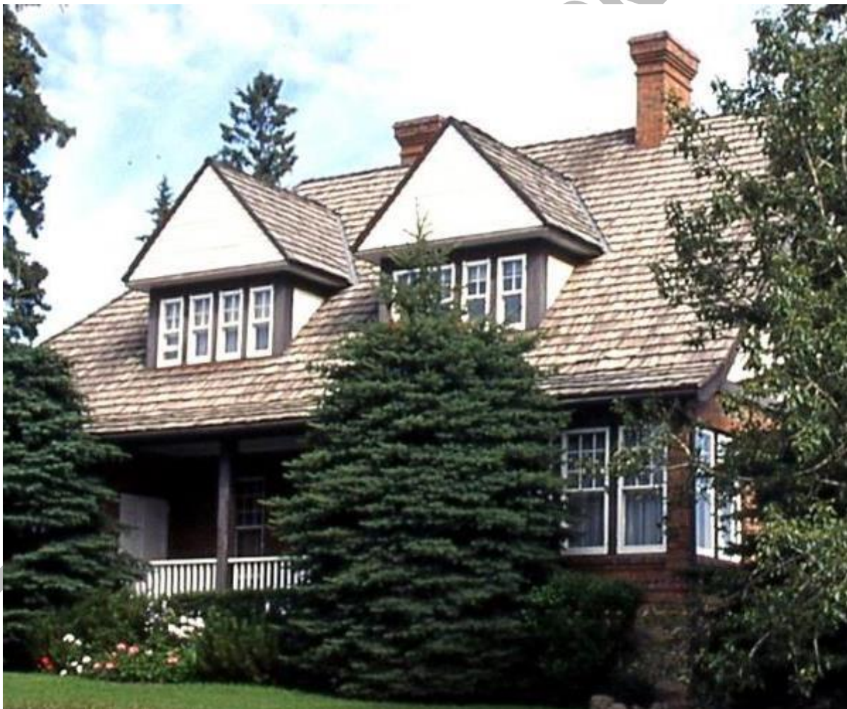
(Image 4.1: South façade ca. 1995 showing side-gable roof with flared bottom eave, inset porch and paired dormers)
