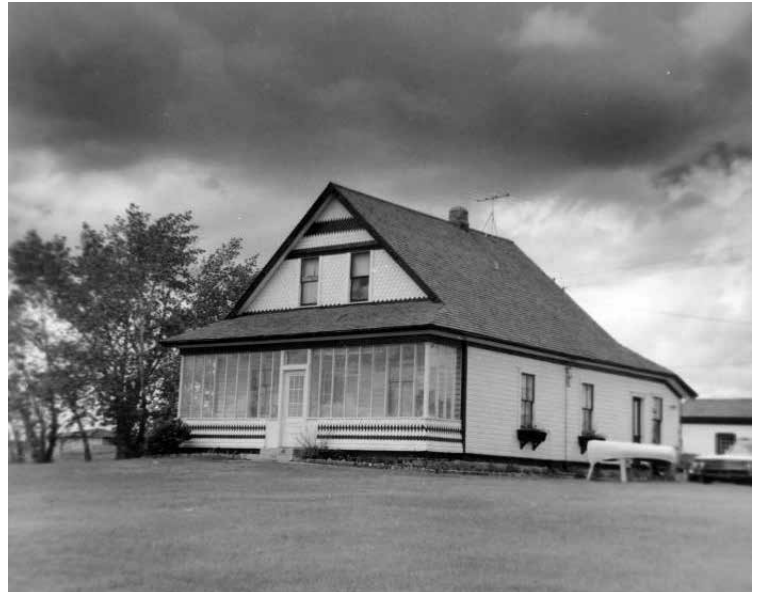
Photo: David D. Oughton residence, 3420–17 Avenue SE. He and his wife Jane and their four sons, homesteaded east of Calgary in the area now known as Albert Park and Forest Lawn. The house was demolished in 1974. Oughton served as town councillor for Forest Lawn and was a trustee for the Bow Valley School Board when it opened the first school in the area in 1906. In addition to farming, Oughton dabbled in ranching and the fledgling oil industry. Before David Oughton’s death in 1956, he donated the Radisson Heights property where Oughton School now stands.
