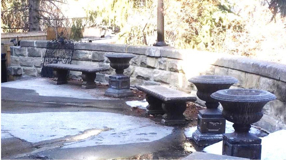
(Image 3.4: Interior of above grade, rounded terrace with cut sandstone balustrade and coping)
