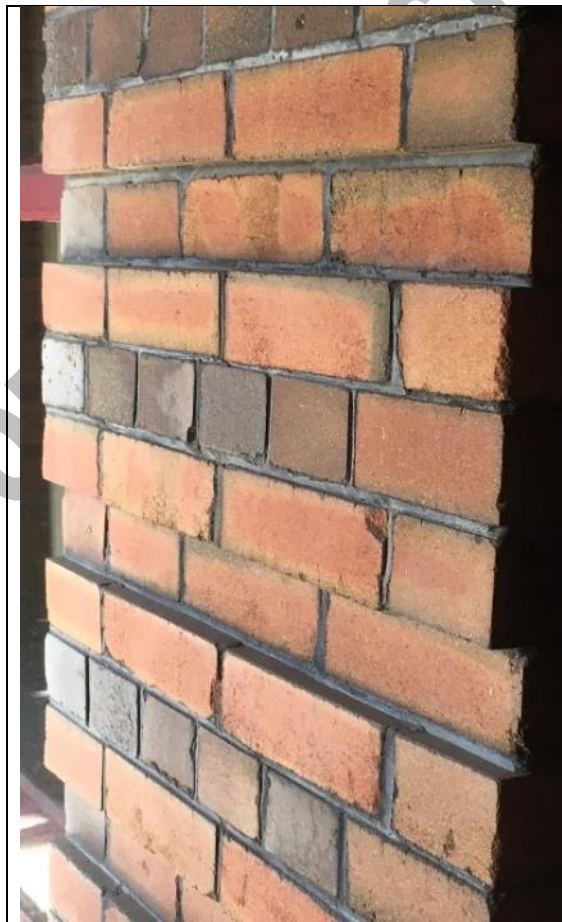
Image 3.5: Detail of red and brown banded, English-bond brick cladding.
