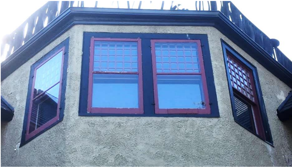
(Image 3.9: Example of original fenestration of multi-light-over-single pane wood windows and casings. Note: Storm windows are not regulated)
