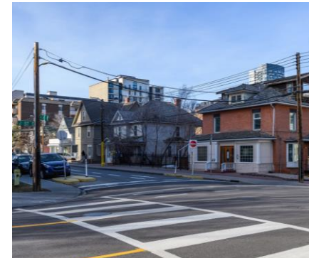
Shallow Utility Relocation Program
