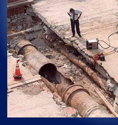
If live about 3km from downtown, changes are the water for your shower arrived in a pipe about this big. A 1.3m pipe has a cross-sectional area of 6,415cm², with ~6,396cm², available for water flow. Ratio of 1.003.
