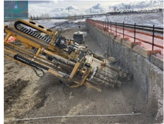
Looking north at the tie back installation work at 78 Avenue Project.
