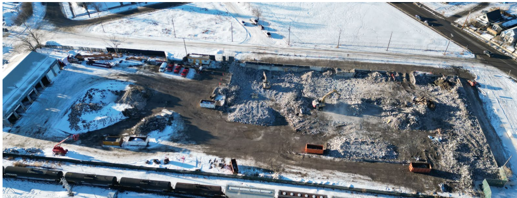
Lilydale demolition site
