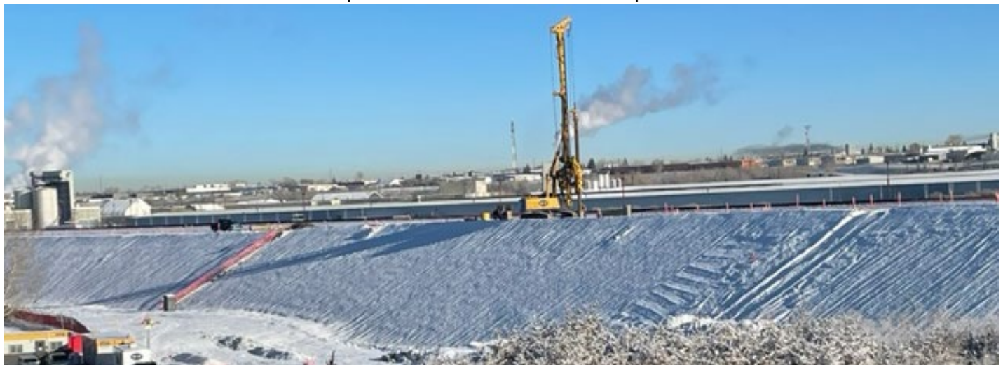
Looking east at the completed 78 Avenue diversion track embankment.
