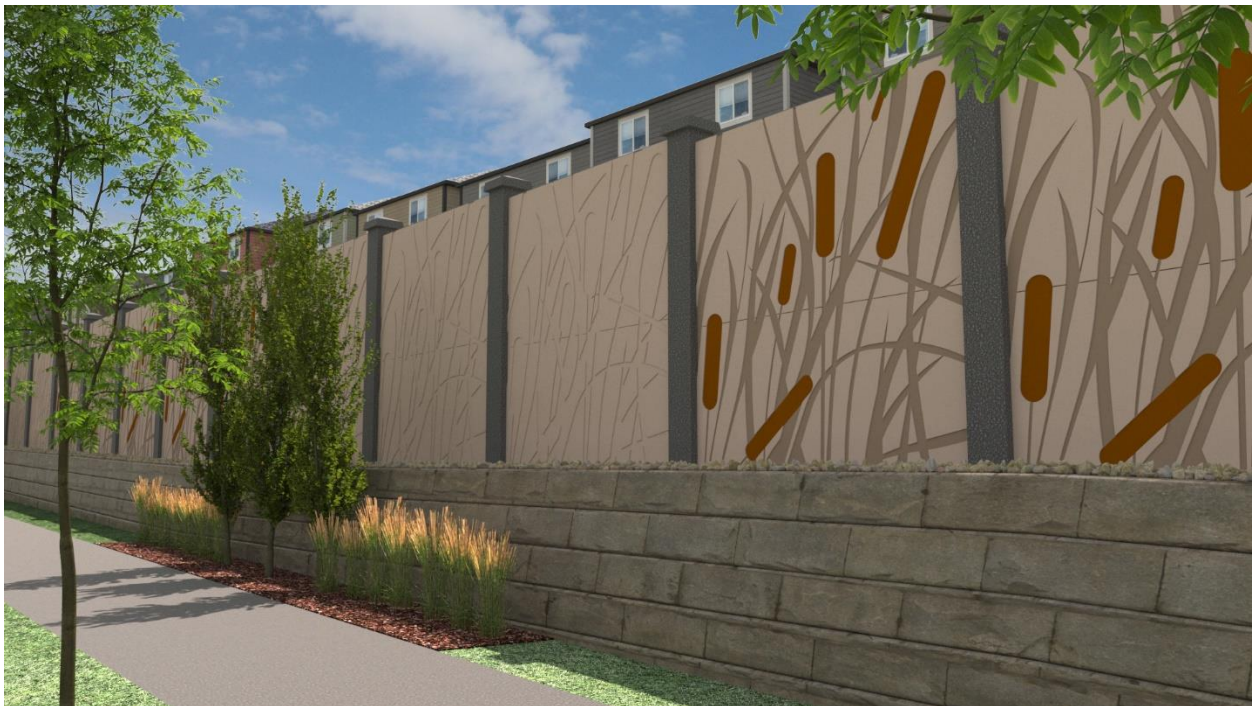
Figure 3: Noise attenuation wall along Evanston homes backing onto 144 Avenue NW
