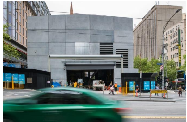
An acoustical shed constructed over an underground station area to minimize noise and dust impacts on adjacent businesses/residences.
