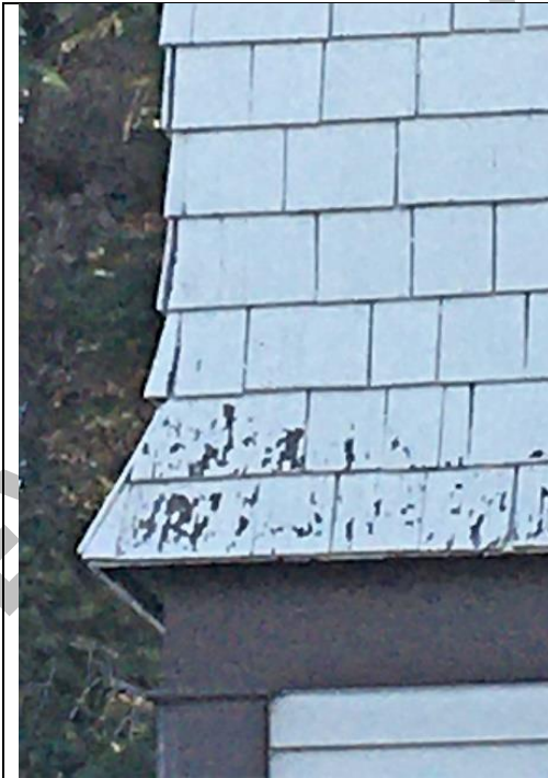
Image 2.6: Detail of flared wood shingled corner on second storey
