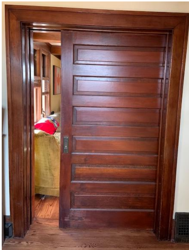
(Image 7.5 Pocket door and example of typical door casing)
