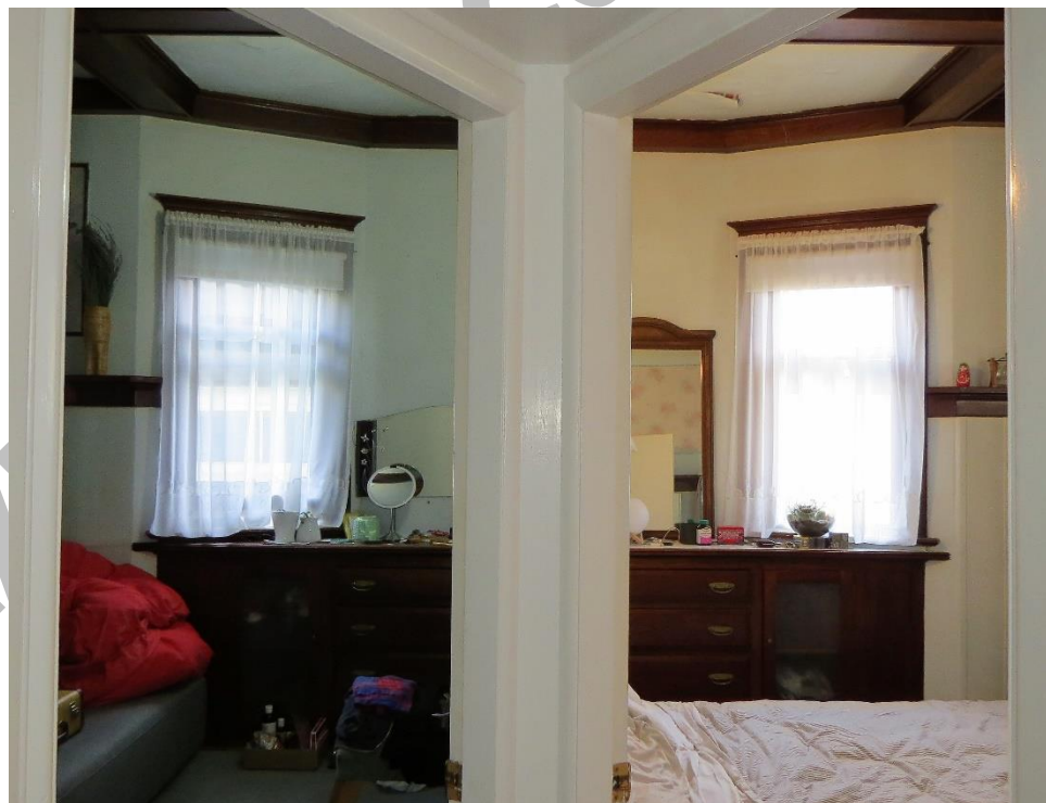
(Image 3.8: Built-in drawers and cabinet (partitioning wall constructed over built-in drawer and cabinet unit during previous renovation))
