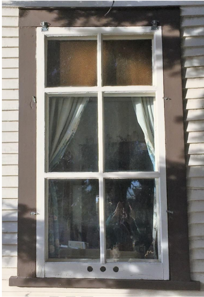
(Image 2.15: Example of 1-over-1 single hung wood window and 6-light wood storm window)
