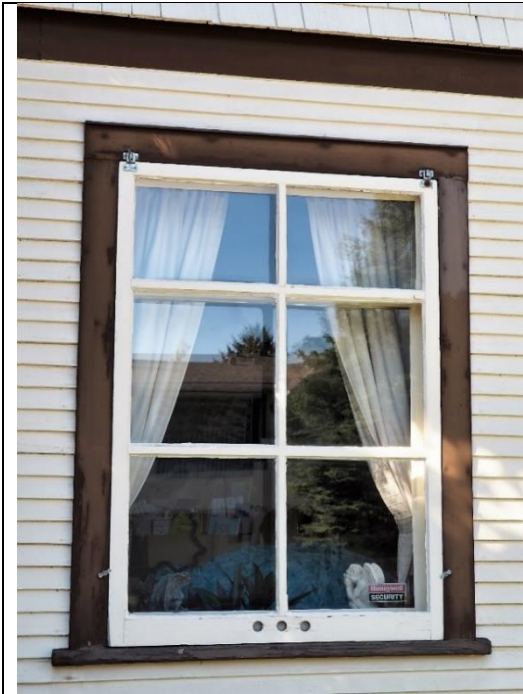
Image 2.11: Example of 1-over-1 single hung wood window and 6-light wood storm window
