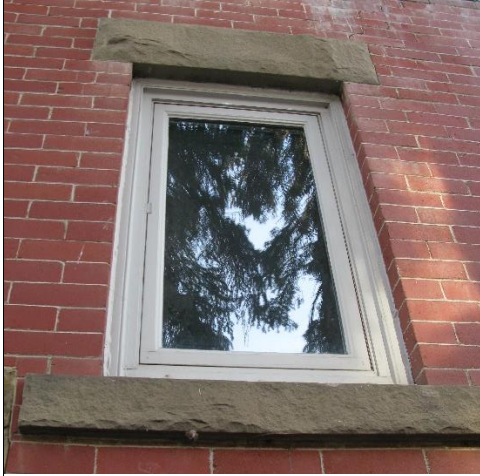
(Image 2.11: Example of window opening with sandstone lintel and sills)
