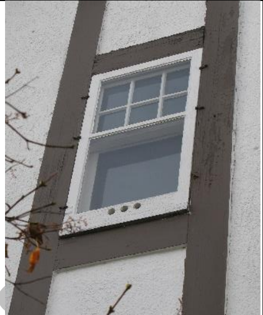
(Image 2.5: example of one of three 6-over-1 wood hung windows with flat heads and painted wood trim)
