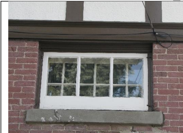
(Image 4.3: 12-pane wood window with concrete sill)
