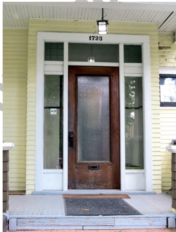
(Image 2.4: Detail of offset front entry on front veranda with side-lights, 3-light transom, wood surround, and original wood door with glazed panel and wood tongue-and-groove ceiling)
