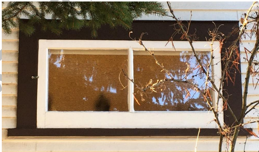
(Image 2.16: Example of fixed one-light wood window with 2-light wood storm window)
