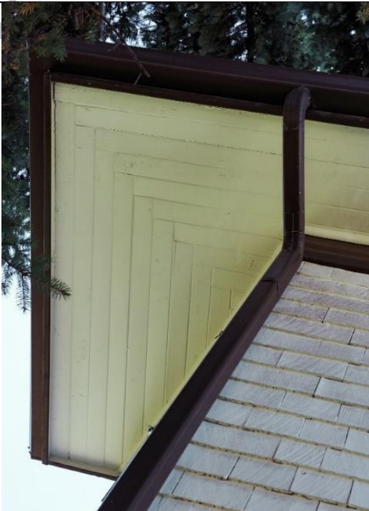
Image 2.7: Detail of closed wood tongue-and-groove soffits under eaves
