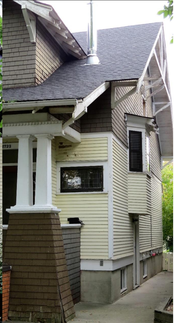
Image 2.6: Shed-roofed bay window with exposed rafter tails on west façade, projecting verges in side gable with stick work in the gable peak, wood belt course, water table with drip mould and corner boards
