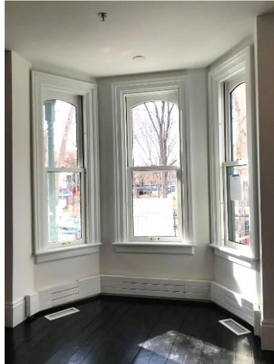
(Image 7.2: Example of window casing)
