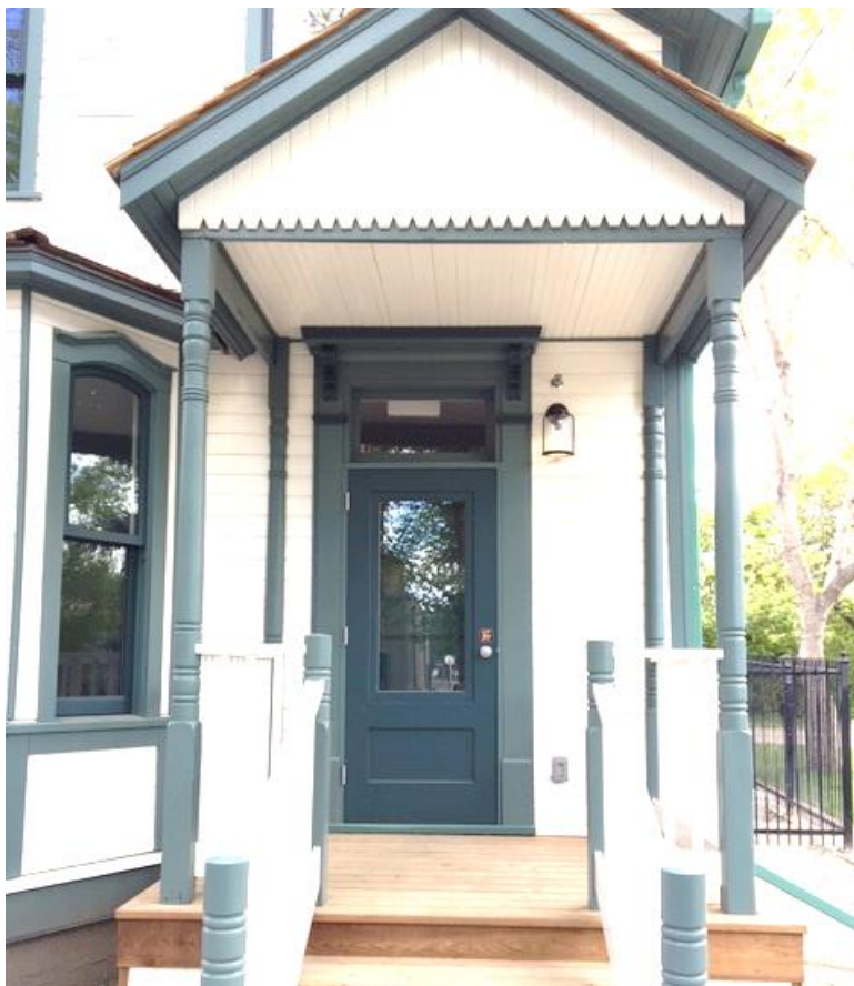
(Image 1.3: Porch and front door surround with decorative crown over single-paned transom)
