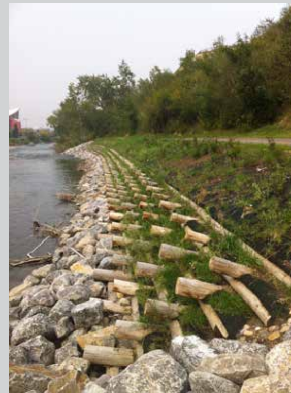
Bioengineering can outperform riprap—the practice of armouring banks with rock.
