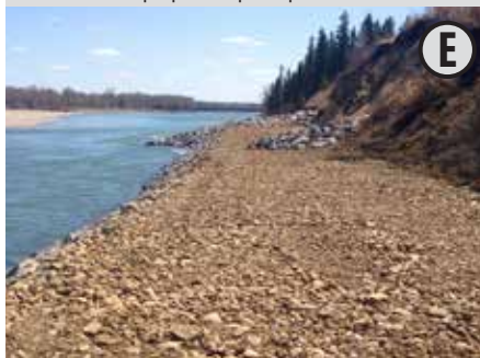
Diamond Cove rip rap and slope toe protection
