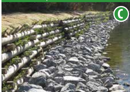
Timber crib wall – upstream of Glenmore Trail
