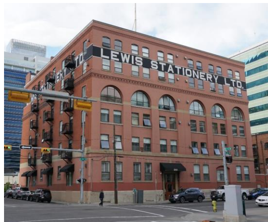
Width doubled in ~1914, "new" east portion wood post and beam; west portion is concrete – little record of design
