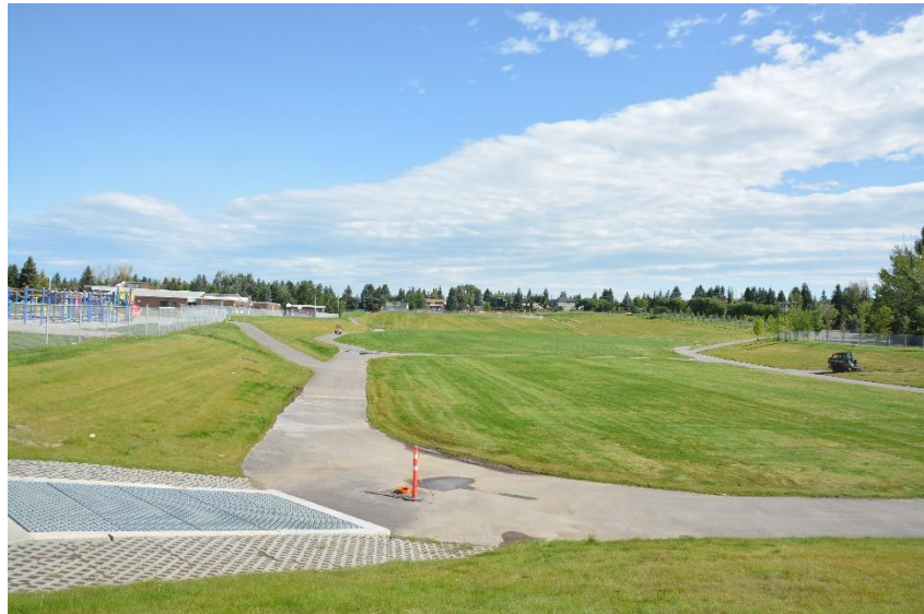
THE BRAESIDE DRY POND WILL ADDRESS FLOODING CAUSED BY RAINFALL IN THE COMMUNITY OF BRAESIDE WHILE ALSO SERVING AS COMMUNITY RECREATION FACILITIES WHEN NOT STORING STORMWATER
